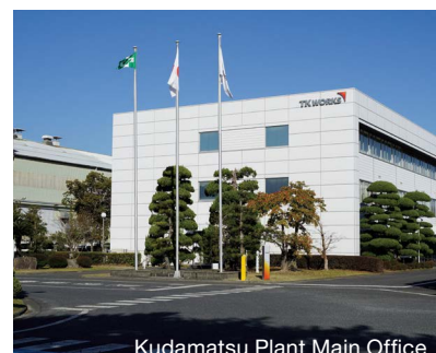
Kudamatsu Plant Main Office
