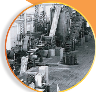
Electrolytic tinning line
