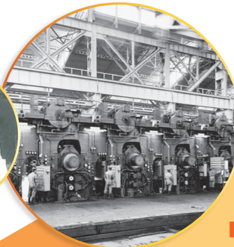
Cold rolling mill
